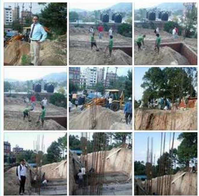
Photos: Kathmandu University School of Law's building construction site at Dhulikhel
